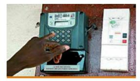
Example of a prepayment meter used for electricity
