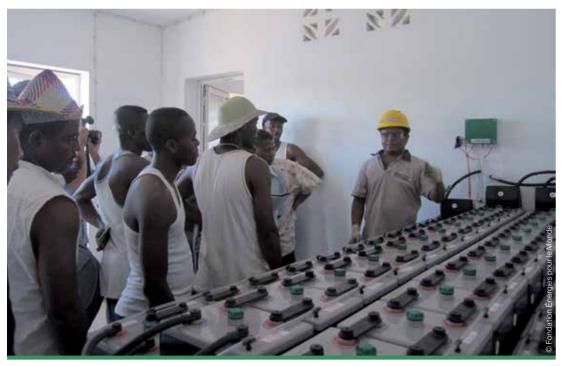
Storage technologies. The batteries of a solar mini power plant in Madagascar
